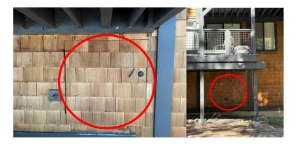
Below is where we would like to cut the access door on our unit. Based on review of our as-built plans, this is the best location structurally and is also the location with the highest interior headroom.
